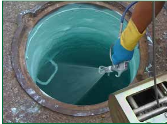
Novocoat SG2500 Lining high build epoxy application.
