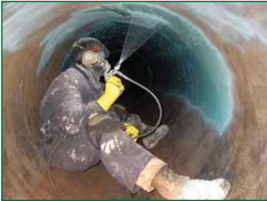
Novocoat SG2500 Lining high build epoxy application.
